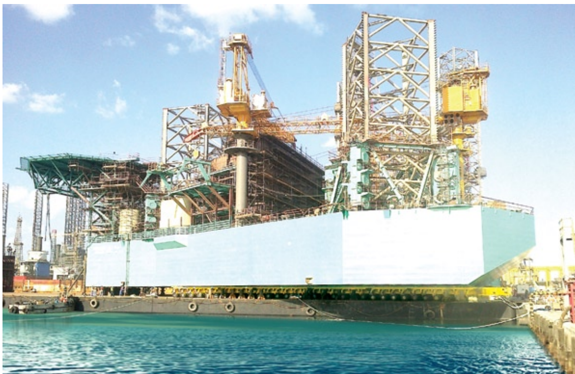
Load out of a 6,300 Te offshore drilling rig onto a semi submersible barge using 232 hydraulic axle lines of self propelled modular trailers (SPMT's).
