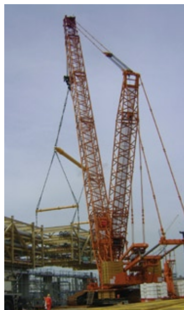
2009 - Erection of a 250 te pre-assembled rack in Singapore using a Liebherr LR 1750
