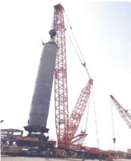
1985 - Erecting an 833 te reactor in Kuwait, a world record at the time.
