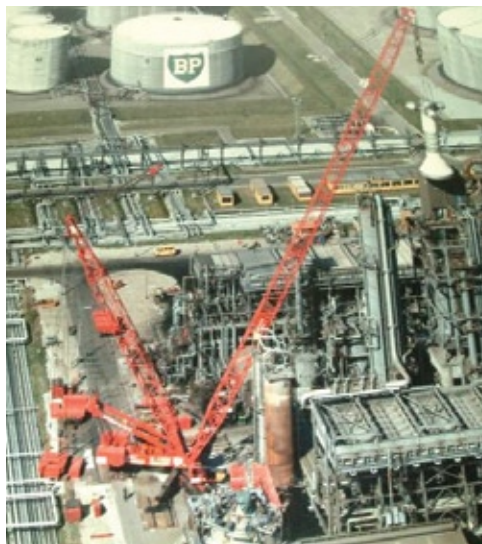
1988 - Lifting a 225 te reactor head in Holland.
