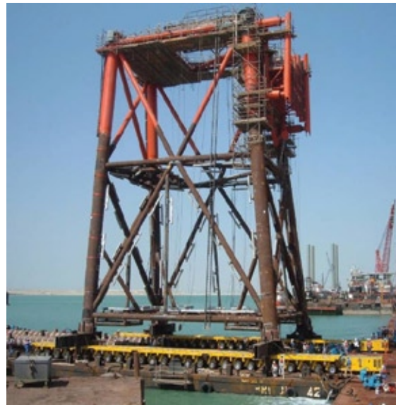
2006 - Load out of a 660 te STD jacket in the U.A.E.
