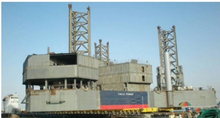
Weighing and load out of a 4,015 te rig hull "Thule Power" onto a barge by means of 154 hydraulic axle lines of self propelled modular trailers (SPMT's).
