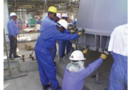
Our surveying team performs checks on foundation holding bolts and vessel orientation prior to lowering onto foundation in accordance with engineering methodology documentation.
