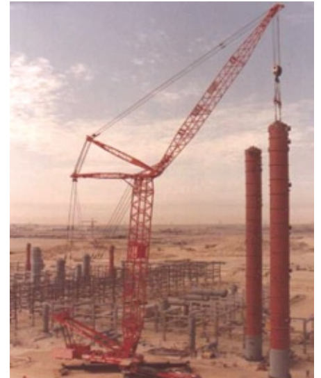
1992-Erecting a 200 te vessel in the K.S.A.
