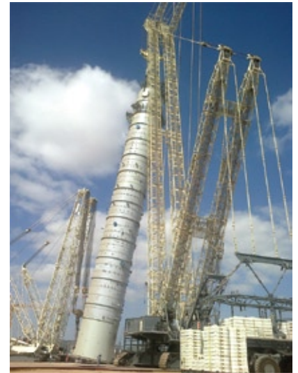
Cranes up to 3,200 te capacity for equipment installation.
