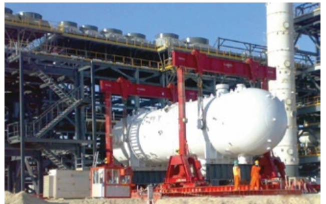
Installation of an HP Separator using a 400te capacity hydraulic gantry system.
