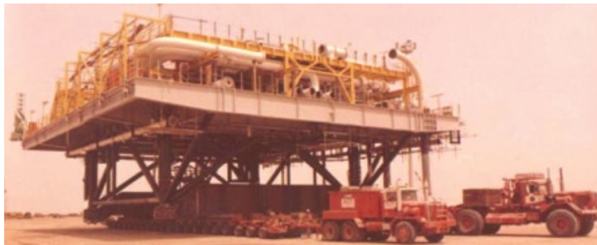
1985 - Transportation & load out of a 210 te offshore module in the U.A.E.
