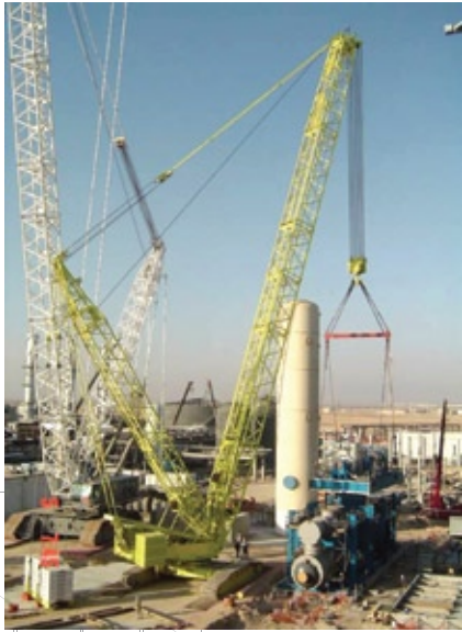
2004 - Lifting a 260 te compressor in Qatar.
